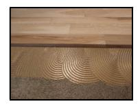
• Allow the laying of parquet on cement screeds with increasing moisture content till 4CM% and save the time needed for laying wooden floors
